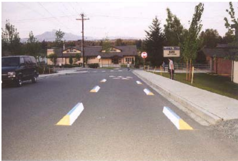
After installation – Lake Stevens, WA (USA)
