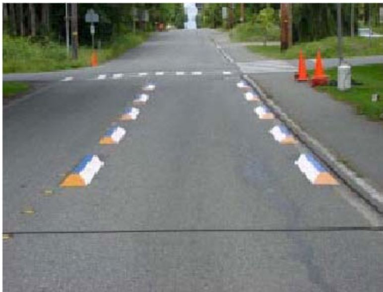
After instalation in Edmonds, WA (U.S.A.)
